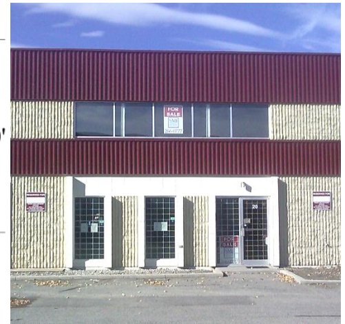
Storefront entrance & 2 nd floor office
